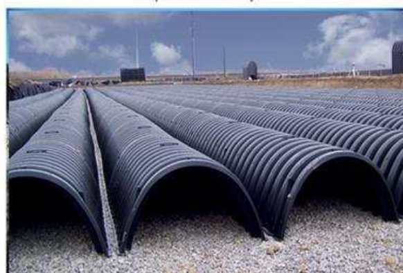
Exemple de Storm Chamber (Source : stormwatercenter)
